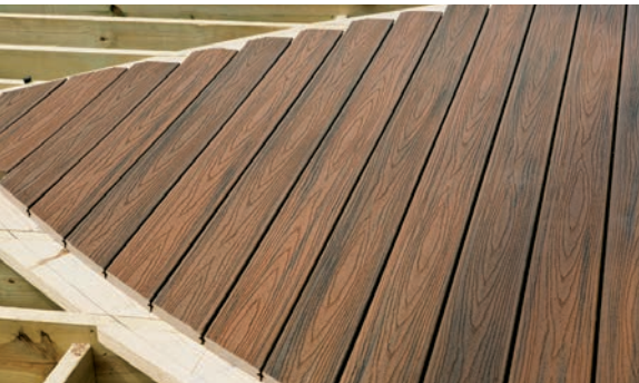
Continue mixing and matching boards to ensure an appealing mix of light and dark tones across the entire deck.
