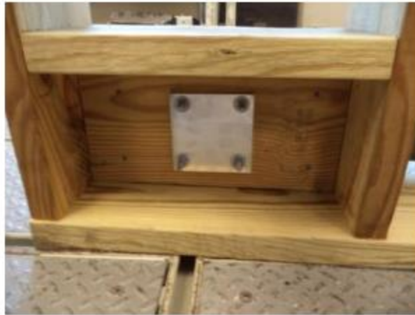
Photo No. 5 Post Mount Installation in Wood Deck - Wood Deck Underside Detail
